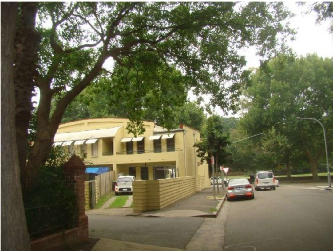
Figure 5. Rear of 2A - 2D Wentworth Park Road from Cowper Street
