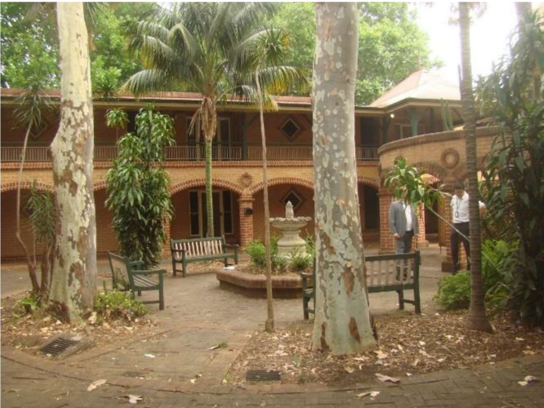
Figure 7. Internal courtyard at 17-31 Cowper Street
